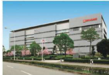
Main Manufacturing Factory
